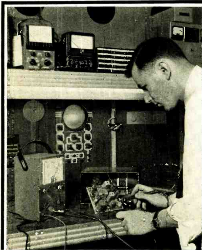
Fig. 2—Measuring leakage with v.t.v.m.
